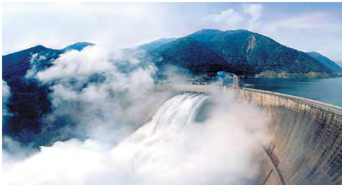
Water sloshing in a reservoir
